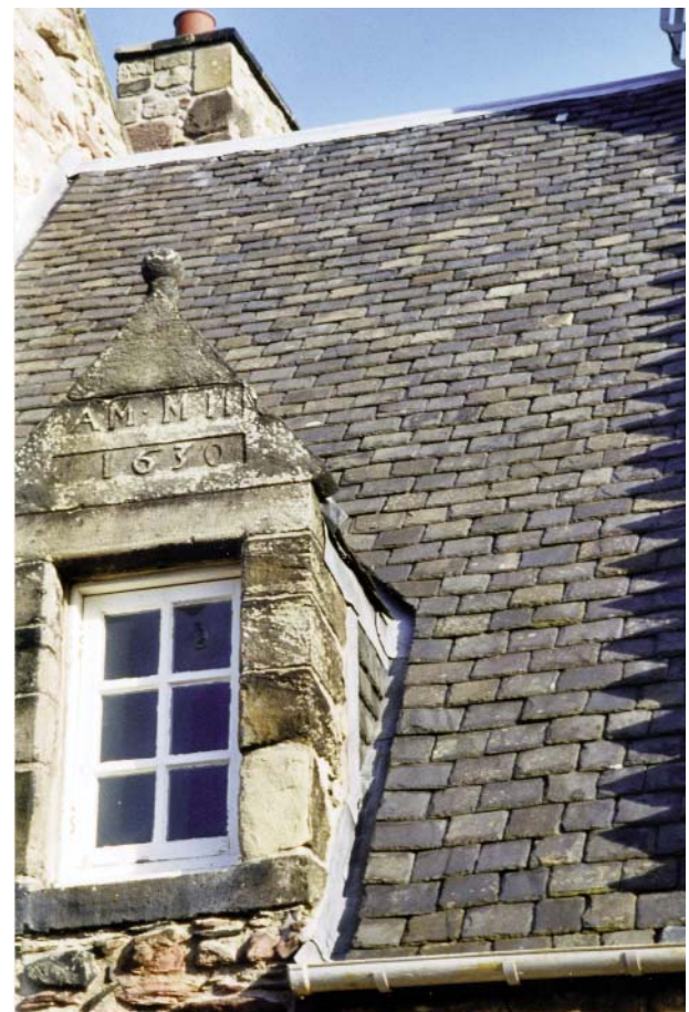
Traditional Scottish Slate Roof, Edinburgh, Scotland
