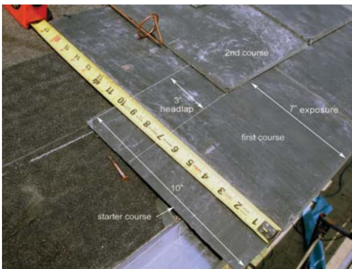
Figure 7: Common mistakes made when installing starter courses include orienting the starter slate face side up, installing no cant, inadequate headlap, and insufficient side-laps. [Photo by Joseph Jenkins]
