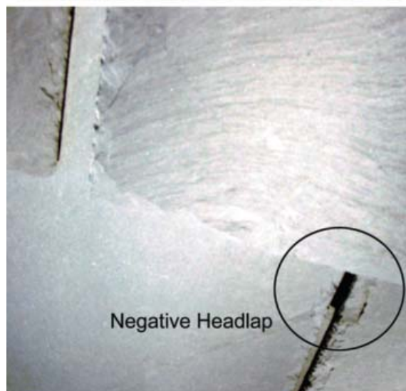
Figure 7: Common mistakes made when installing starter courses include orienting the starter slate face side up, installing no cant, inadequate headlap, and insufficient side-laps. [Photo by Joseph Jenkins]
