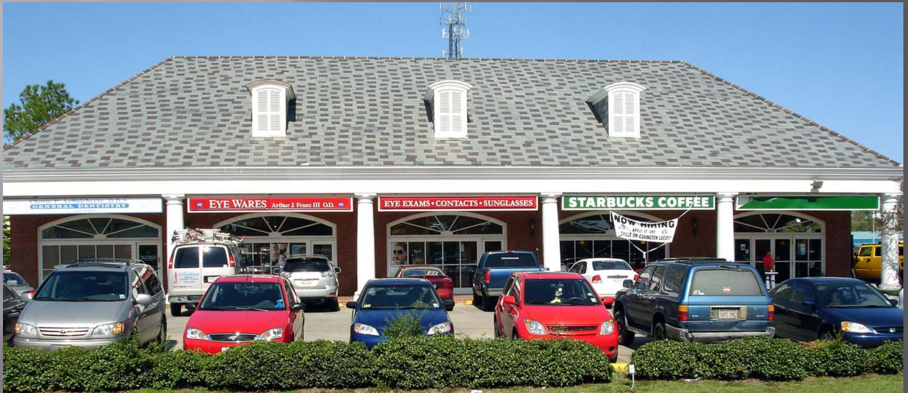
Lack of headlap caused this roof to be condemned.
