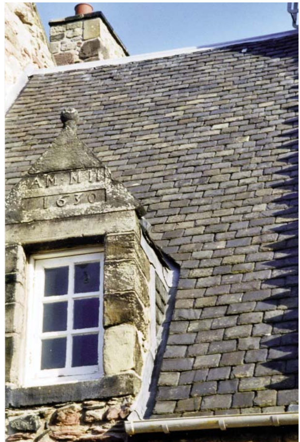
Traditional Scottish Slate Roof, Edinburgh, Scotland
