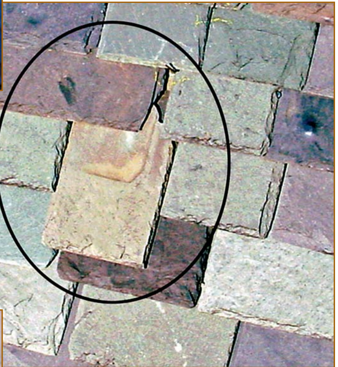
Figure 16 – This slate was nailed so tightly that the nails broke through the slate and the slate is now sliding out of place.
