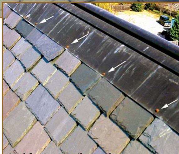
Figure 28 – Metal fasteners should always be compatible with the metal they are fastening. Steel fasteners on copper, as shown, will deteriorate.
