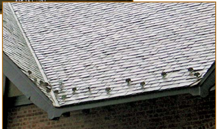
Figure 31 – Snowguards must be installed in adequate quantities, or they will get knocked off in the first bad ice storm, damaging the roof in the process.
