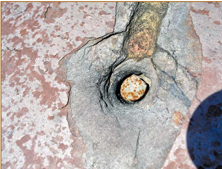
Figure 15 – A protruding nailhead can eventually wear a hole in the overlying slate.
