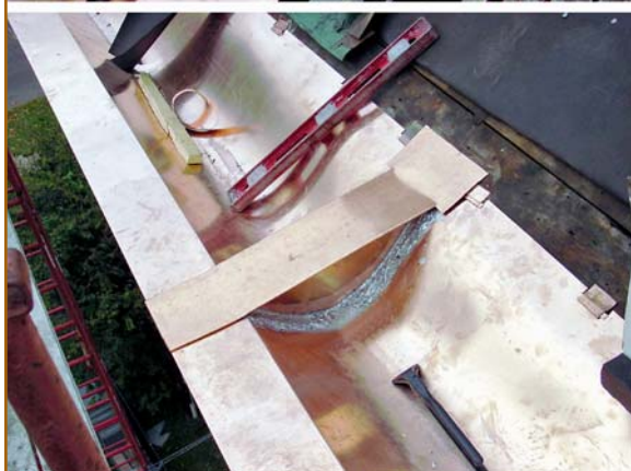
Figure 27 – Expansion joints allow built-in gutters to move when expanding and contracting, thereby relieving the stress on the solder joints and prolonging the life of the gutter.
