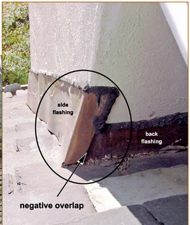
Figure 22 (left) – Chimney corner flashings should be either folded or soldered. If neither is evident, then the corner is either sealed with sealant or not at all. In either case, this is a leak waiting to happen.
