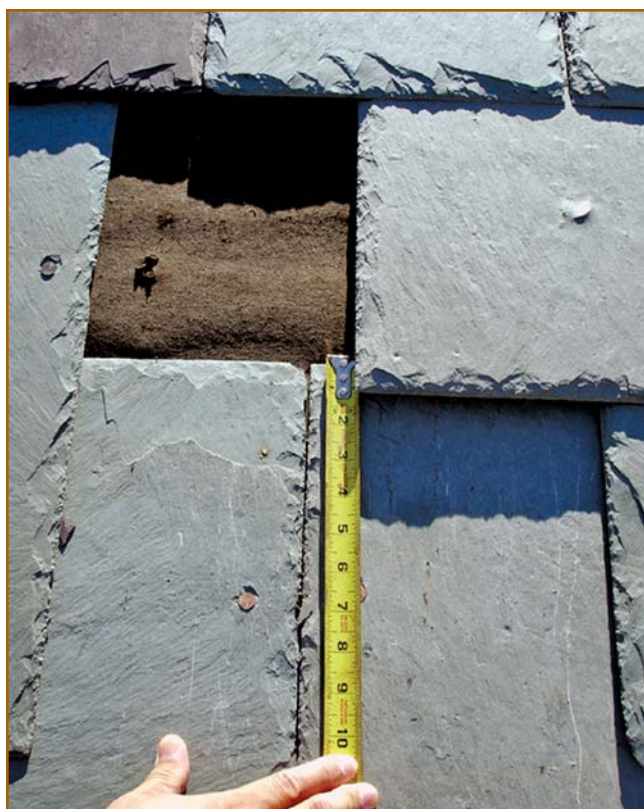
Figure 10 – This is an example of inadequate headlap on a shopping center roof in Louisiana.
