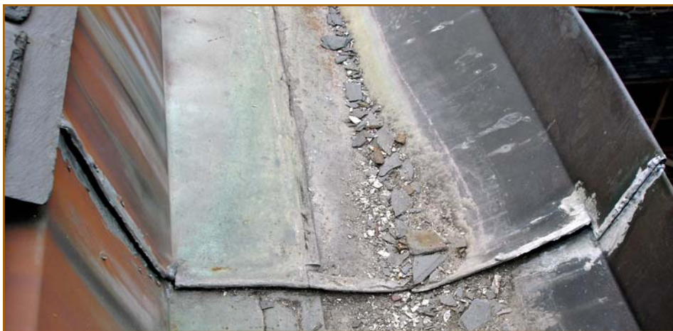
Figure 25 – This is a perfect example of a new built-in gutter showing failed solder joints because not a single expansion joint was installed in the gutter system.
