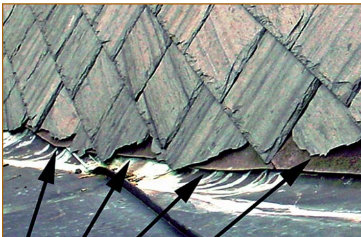
Figure 33 – Slate roofing requires the correct tools to do the job right. There is no excuse for the sort of work shown here.
