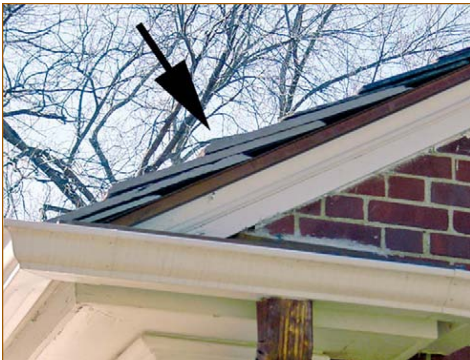
Figure 32 – Diamond blades cut a square edge on slates, making them stick out like a sore thumb.
