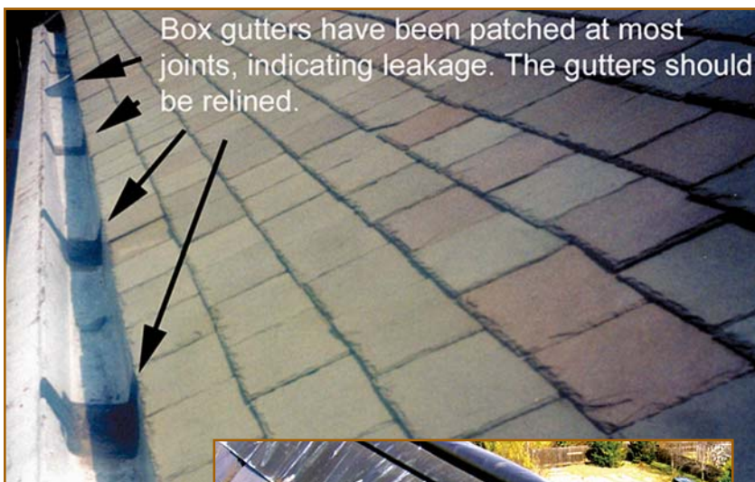
Figure 26 (above) – Box gutters have been patched at most joints, indicating leakage. The gutters should be relined.
