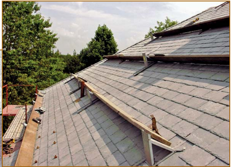
Figure 19 – A correctly staged slate roof will enable roofers to install the slate without needing to walk on the shingles.
