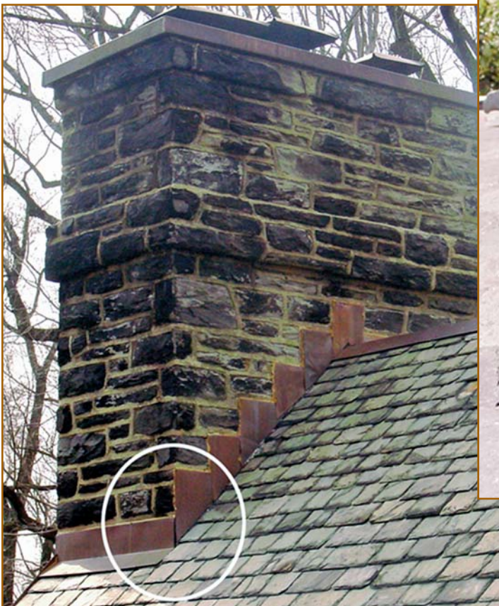
Figure 22 (left) – Chimney corner flashings should be either folded or soldered. If neither is evident, then the corner is either sealed with sealant or not at all. In either case, this is a leak waiting to happen.
