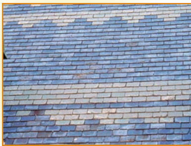
Photo 3: Pennsylvania black and Vermont unfading green slate, 120 years old, on St. Andrews Cathedral. Black is worn out; green is still good.
