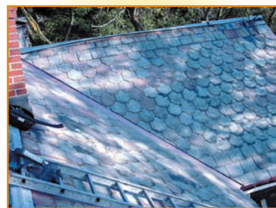
Photos 4, 5, and 6: Typical flashing repair – before, during, and after: valley replacement on badly abused residential slate roof.
