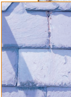
Photos 10, 11, and 12: Typical bad repairs. 10: wrong type and shape of replacement slate, face-nailed through overlying slates; ugly and a sure leak. 11: Nail in slot to fasten replacement slate, then caulked – another sure leak (should have used a bib flashing). 12: Nail in slot without caulk or bib flashing becomes a “hidden leak” because the hole is almost invisible.
