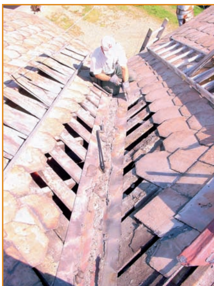
Photo 9: Barn roof showing lath roof decking. 100-year-old white oak lath is still in good condition despite the totally deteriorated valley flashing.
