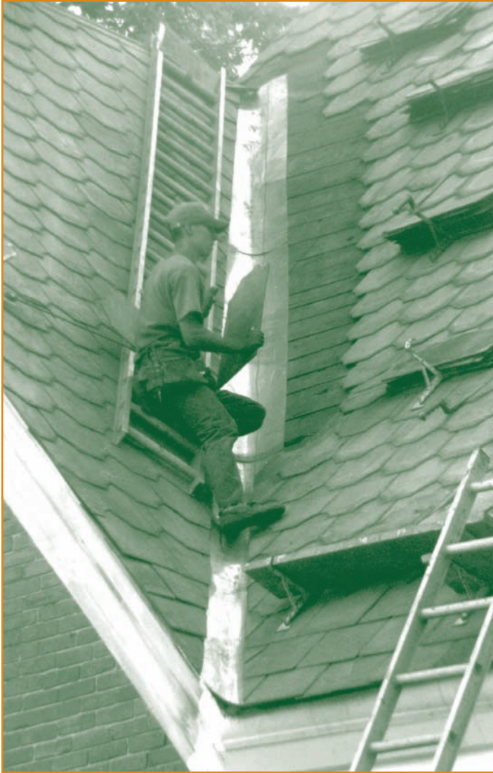
Photo 14: A fully sheathed board roof deck with a temporary 30-lb. felt underlayment is a very successful tried and proven roofing system used with slate roofs and should be used with all new slate roofs for best results. The felt is optional. No underlayment is needed for the proper functioning of the roof. The valley replacement on a 104-year-old church shown above reveals the 1" hemlock board decking and the complete absence of underlayment. The slate is PA black, still in good condition. No water can penetrate the slate/copper roof system, which is why the underlayment is optional.
