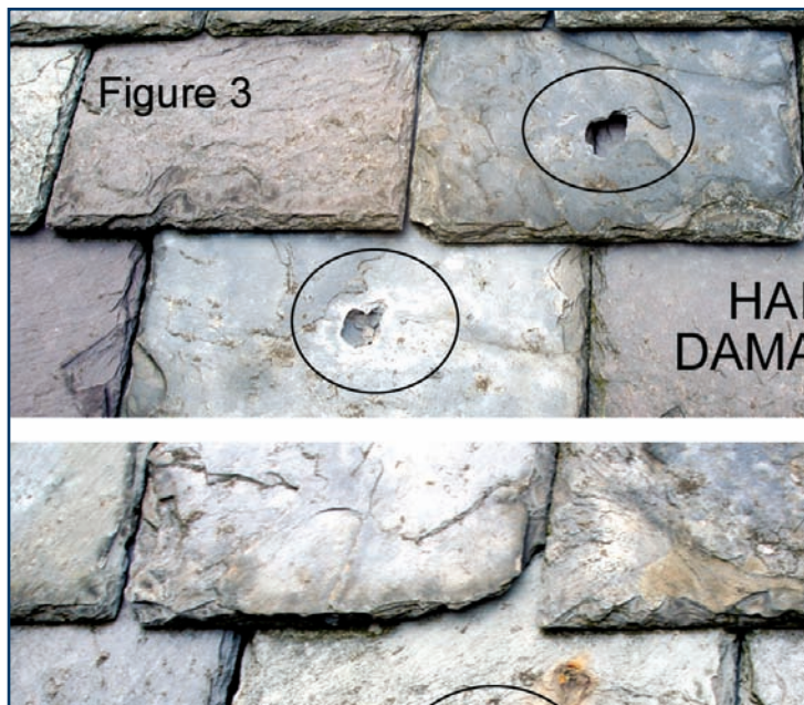
Figure 3 – Hail-perforated slates should simply be removed and replaced. Hail damage rarely justifies replacement of an entire slate roof.
